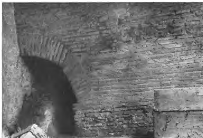
Fig. 232 — S. Maria in Cosmedin. exterior of north wall of left aisle; remains of earlier niche (Photo: Corbett).
